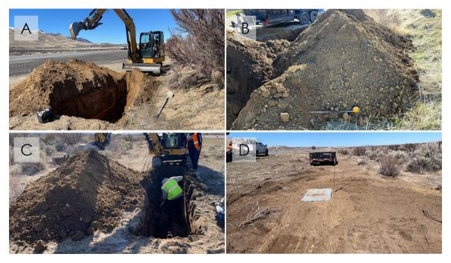
Figure 8. Examples of ground disturbing activities in Lassen County for February 2025: (A) vault excavating at L-27.6, facing northwest; (B) excavation spoils from L-26.2, facing east; (C) vault excavating at L-27.2, facing southwest; (D) completed and backfilled vault excavation at L-27.2, facing northwest.
